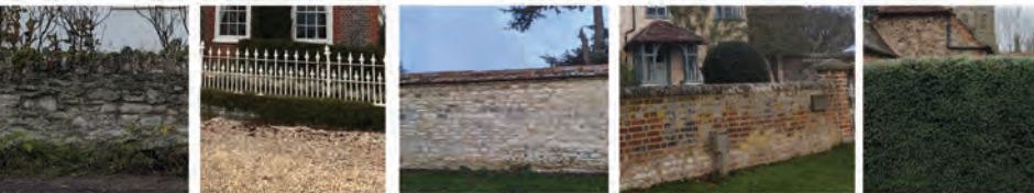
Uncoursed rubble stone wall boundary with stone coping Low brick wall topped with railings Local coursed stone / clunch wall boundary with clay tile capping Mid height frontage brick wall boundary with half round brick coping Hedged front boundary
