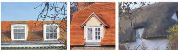
Small cottage casement dormer windows, generally set into the roof with some cutting of the eaves line. Simple form detailing or decorative bargeboards. Dormer windows are small, non dominant features
